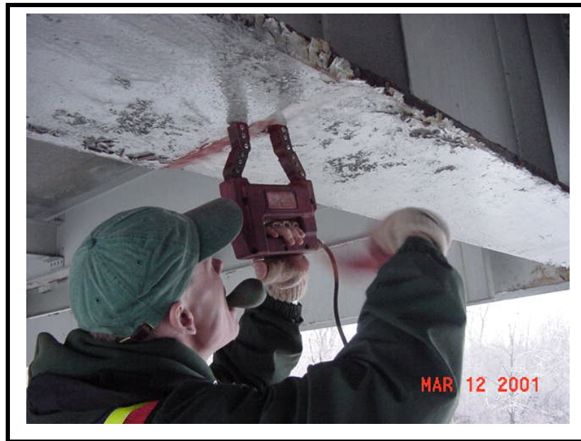
Figure 6:16-3: Magnetic Particle Testing on a Built-Up Plate Bridge Girder Butt Weld
