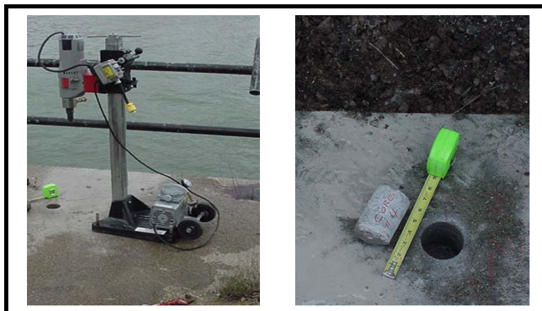
Figure 6:13-1: Concrete Coring Machine (Left) and Core Sample (Right)
