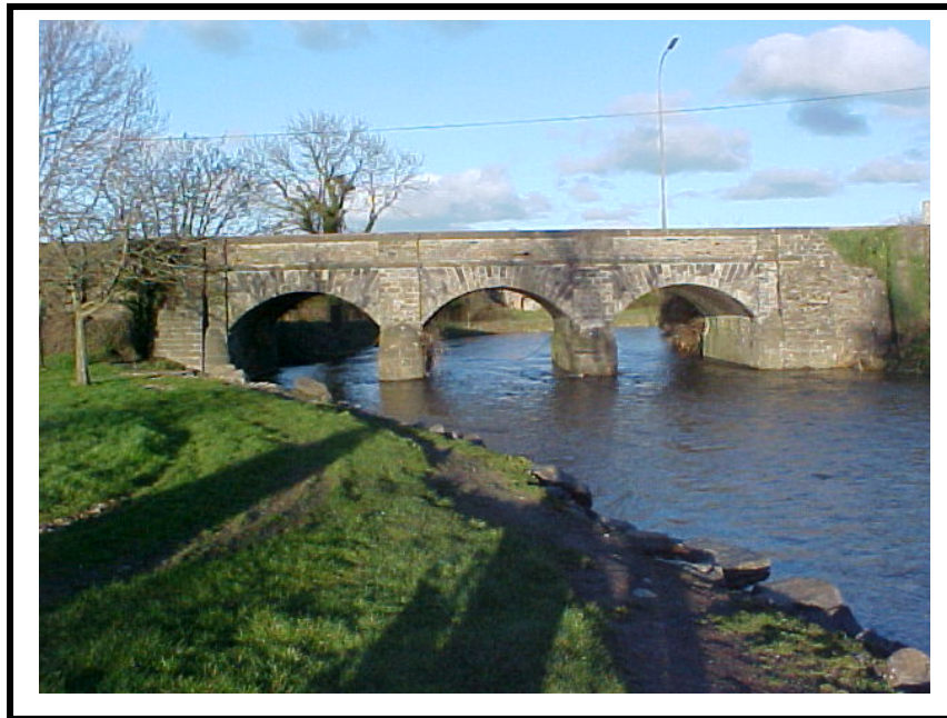
Figure 6:18-1: Bridge With Unknown Foundations
