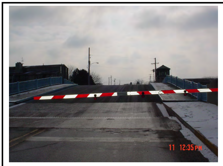
Figure 5:1-3: Franklin Street Bridge in Partially Open Position
