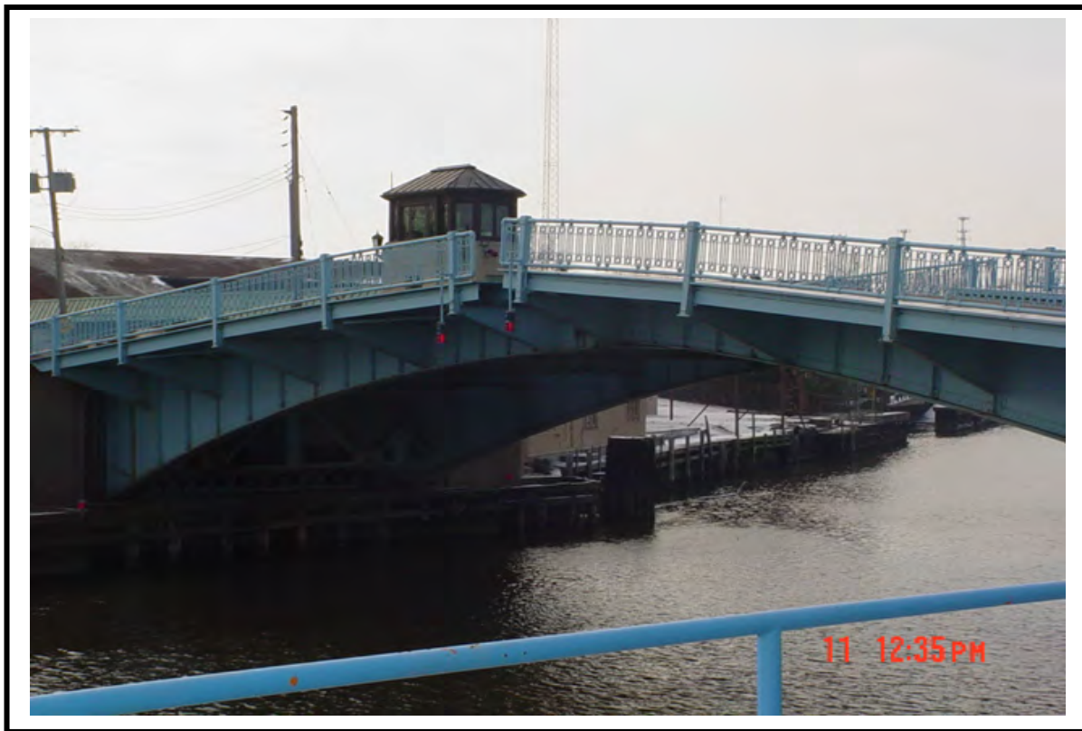
Figure 5:2-1: Franklin Street Rolling Lift Bridge
