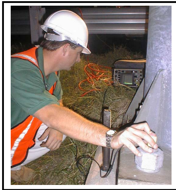
Figure 6:14-4: Inspector Conducting Ultrasonic Testing on a Sign Structure Anchor Bolt
