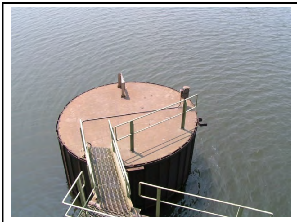
Figure 5:2-4: Dickey Road Pier Protection Cell
