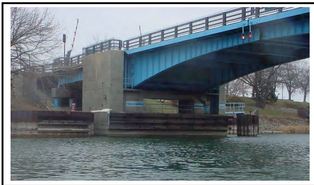
Figure 5-1-4: Movable Bridge Span Accessible From the Bank
