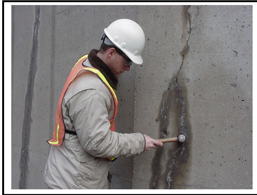
Figure 6:3-1: Inspector Hammer Sounding a Bridge Abutment
