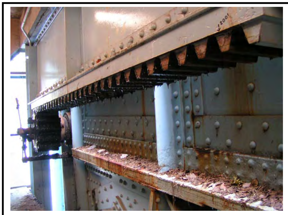
Figure 5:2-2: Rolling Lift Bridge Teeth
