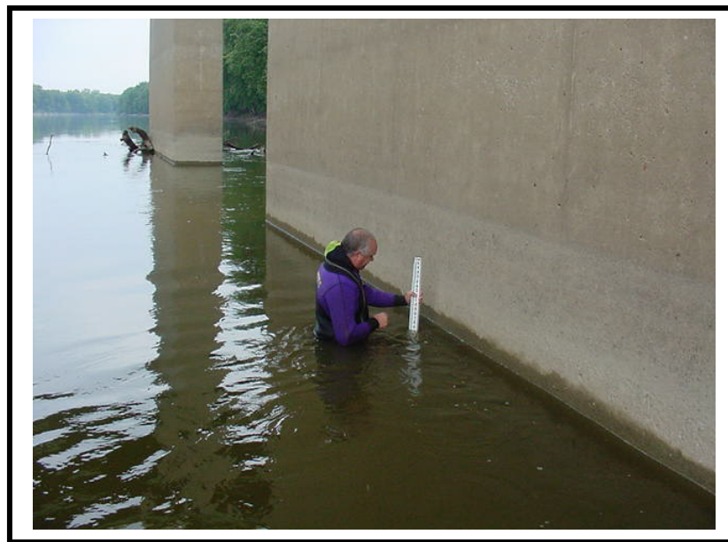
Figure 6:19-1: Inspector Using a Sounding/Range Pole
