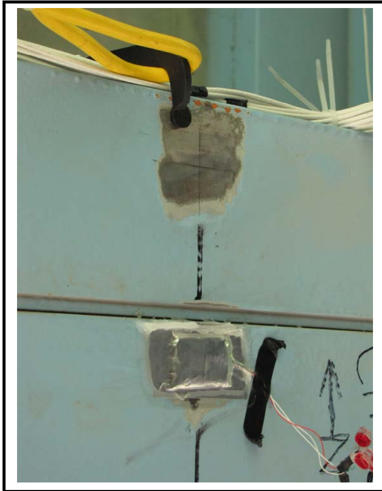
Figure 6:17-5: Strain Gauge Close-Up
